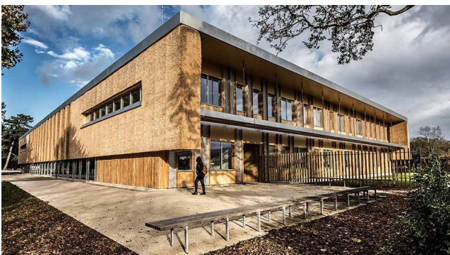
Figure 1.13 - The Enterprise Centre Source: Architype
