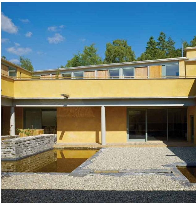
WISE Building External view
